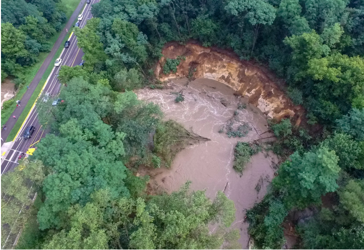
Pheasant Branch Creek Bank erosion east of Park St looking north
