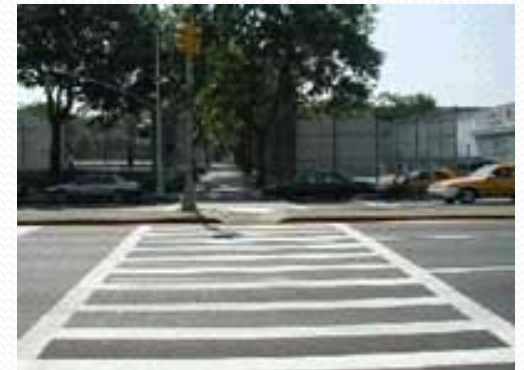
Ladder Type Markings
