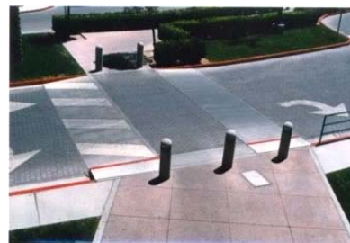
Raised Pedestrian Crossing Salt Lake Airport Source: ITE Pedestrian Bicycle Council
