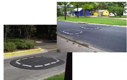
Speed Cushion Source: ITE Pedestrian Bicycle Council
